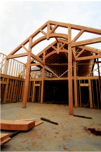
A structural Douglas Fir Timber Frame going up. For scale, the posts are 12x12s.
